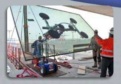
The MAVLift 1320 Offroad is the largest electric model in the off-road series. Built with smooth precision controls, the MAVLift 1320 is great for serious glaziers installing heavy duty commercial glass.
