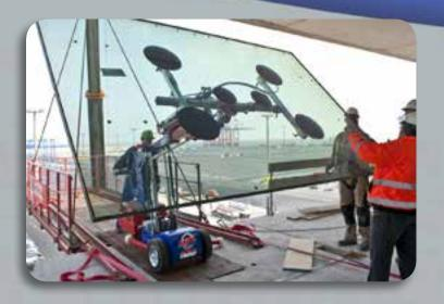
The MAVLift 1320 Off-Road is the largest electric model in the indoor series. Built with smooth precision controls, the MAVLift 1320 is great for serious glaziers installing heavy duty commercial glass.
